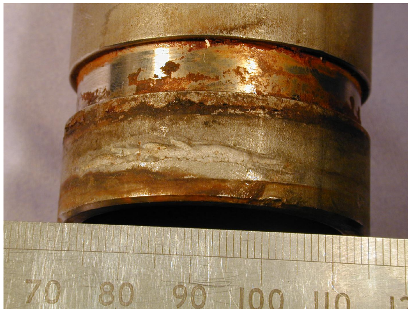
FIGURE 4 - Crevice corrosion of 316L at high pressure pipe joint.
